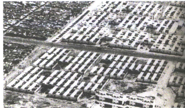
FIG 1.2: AERIAL PHOTO OF CARRIÈRES CENTRALES MASS HOUSING PROJECT, 1955
